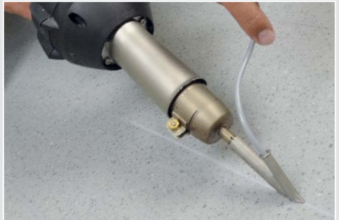
Plastic and linoleum floors
