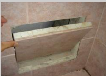
Step 3 – Slot panel to frame
