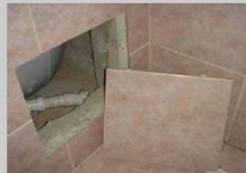
step 2 – Bond tile on to panel
