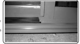
4-On top of the interlock, lift the Top fix block to touch the Head frame.
