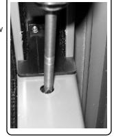
6-On bottom of the interlock, use screws (12X8) to secure bottom interlock to the sill both inside & outside.
