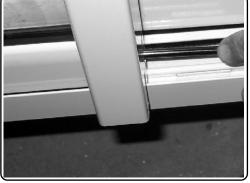
6- Place the sliding panel"B" into frame in the middle track.
