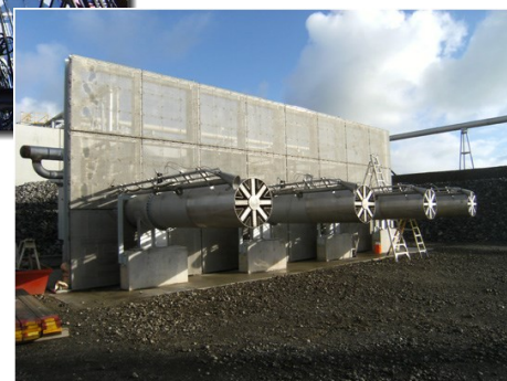
Ladder Heatshields protecting processing piping in KUPE GAS onshore 'Burn Pit'
