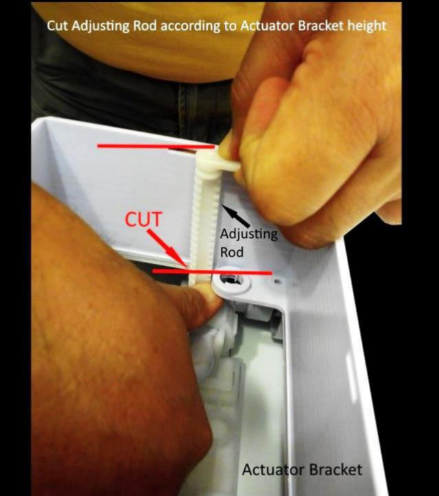
Step 3 (cont'd): Install the Adjusting Rod onto Actuator
