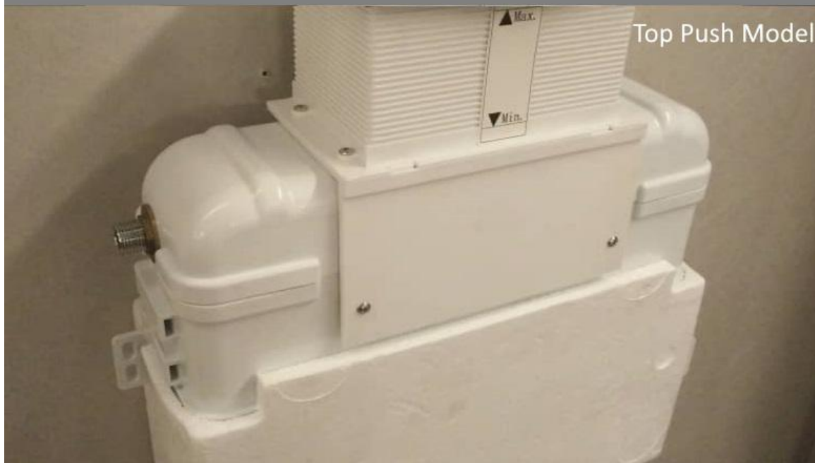
Affix Actuator Box & Temporary Cover
