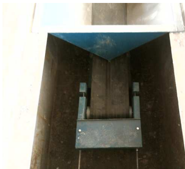
Belt Conveyor Floor recovery
