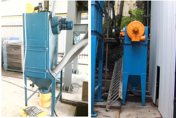
Abrasive Cleaning Dust Collectors Installation
