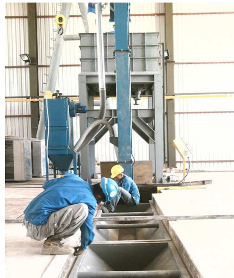
Recovery Floor Hopper & later installed with heavy duty grating is applicable to both belt conveyor or screw conveyor systems
