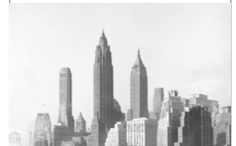
Carrier announced that the four biggest and most modern post-war skyscrapers in New York city would be air-conditioned from top to bottom by Carrier's Conduit Weather Master System.
