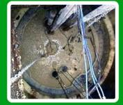
BEFORE TREATMENT: Grease Cap Thickness = 8 inches Grease Blanket = 100% Cover Grease = Compact Cleanout Cycle = 25 - 30 days
