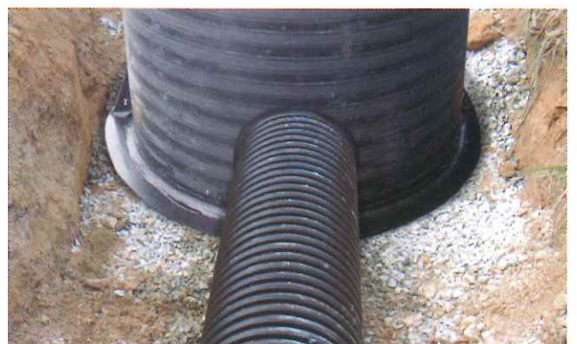
Connection of WEIDA DWCP to Floline 3-W manhole
