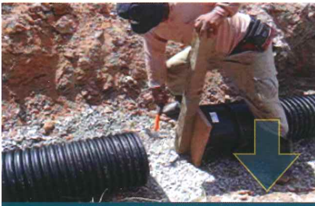
Pipe is pushed into the socket to complete the connection
