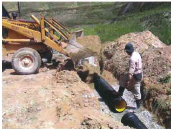
Backfilling of sewer pipe
