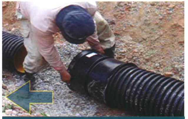
Align and insert socket into pipe
