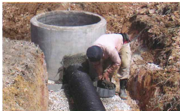
Grouting WEIDA DWCP to a concrete manhole
