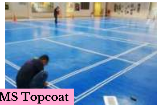
Mortal Epoxy Water Proofing Primer 5mm + PU MS Topcoat 3mm for Sony Factory
