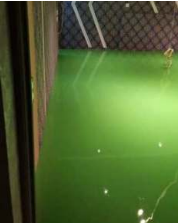
Epoxy Metallic Self Leveling System
