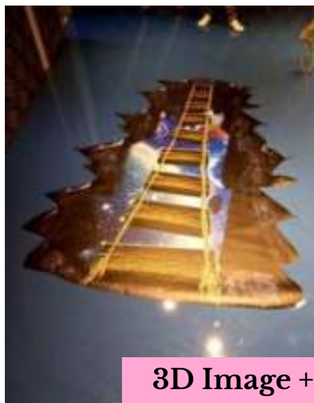
3D Image + Self Leveling Epoxy + PU UV Topcoat
