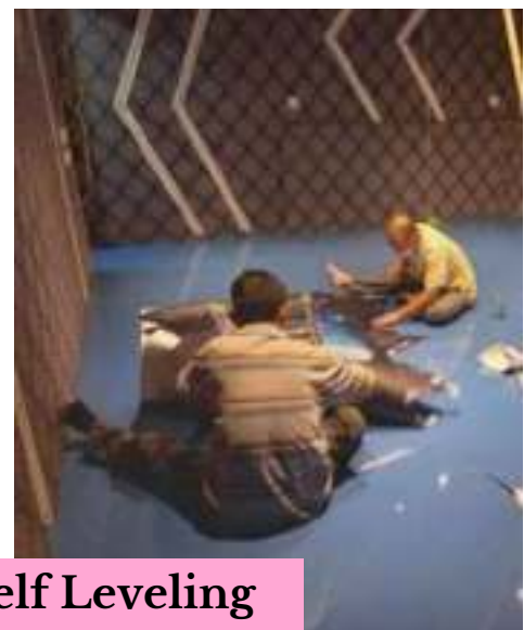
3D Image + Self Leveling Epoxy + PU UV Topcoat
