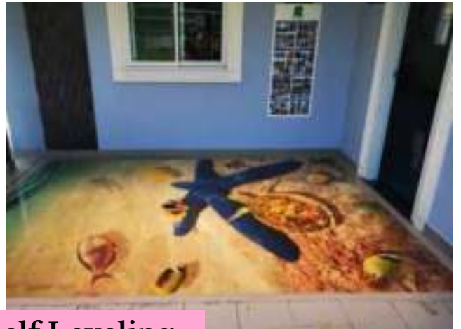
3D Image + Self Leveling Epoxy + PU UV Topcoat
