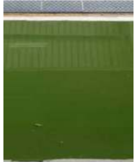
Mortar + PU MS for Loading Bay
