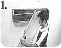
1.First open the Open type cleaning cover and make sure the white connector in the middle are connected and fixed.
