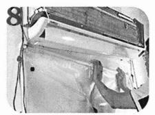
8.Insert the transparent film to the lower back of the air conditioner.
