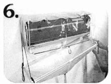
6.Pull up open type cleaning cover's two rope stoppers that is against the wall until it's near the bottom of the air conditioner on both side.
