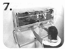
7. Must remember to leave a gap for you to insert the transparent film in the back of the air conditioner.
