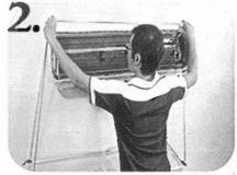
2.Use both hands to pull up the bracket and hanging above the split type air conditioner on both corners, must insert and securely fix the plastic board (Push button) in the back of the air conditioner.
