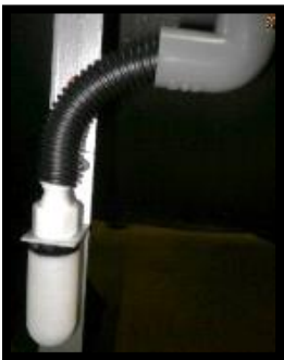
Sampling Point (Leak Detection Point)
