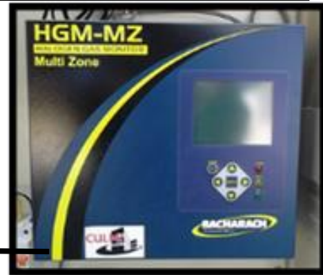
Bacharach Gas Monitor HGM-MZ-12-Zone (S/No : 15120434)
